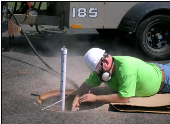
**2** After sandblasting, blast the surface with clean air to remove any loose sand that may have been deposited onto the surface. The substrate surface **MUST** be dry and be free of loose sand.
