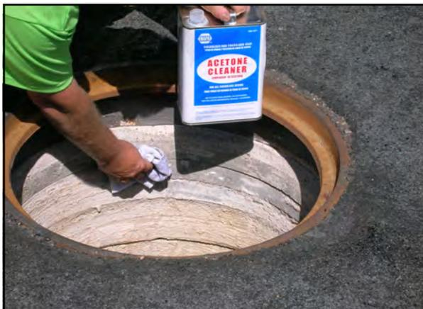
**3** When air blasting is finished, an acetone wet wipe of the entire surface to be coated is recommended. This is to get a mechanical wipe of the surface, a wet wipe of the surface and a high flash point wipe of cementitious portion of the surface to evaporate any surface moisture in the non metallic portion of the chimney area to be coated with Flex-Seal Utility Sealant.
